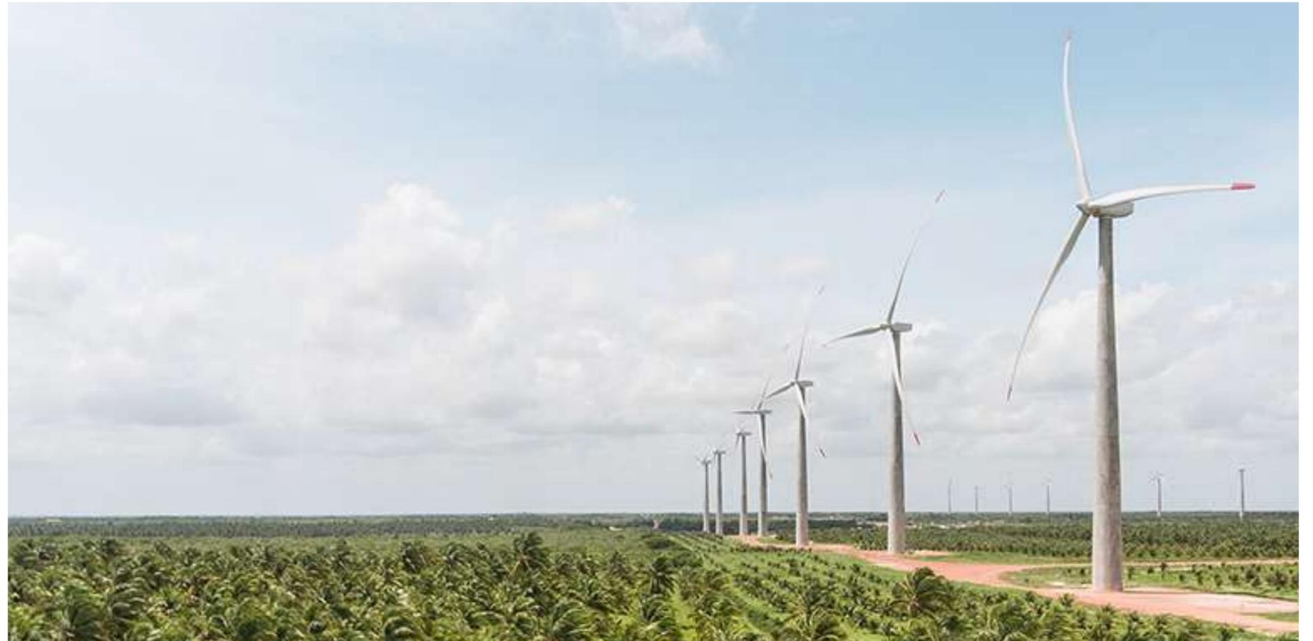
Located in the municipality of Itarema (CE), the wind farm consists of 69 wind turbines and has an **installed capacity of 207 MW**. The energy produced is transported by a 26.5 km transmission line to the substation located in the municipality of Acaraú (CE), where it is connected to the National Interconnected System (SIN) network.
